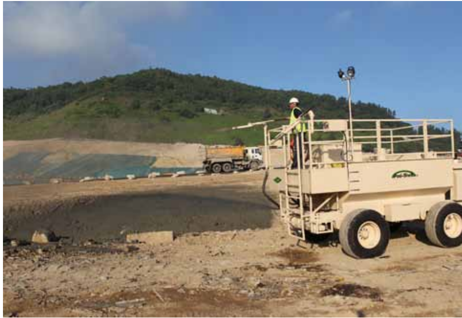
Erosion Control in Hong Kong, using PSA-2000 Applicator
