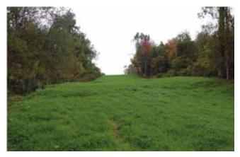
Figure 2. EQT pipeline project in Alleghany County, Pennslyvania, on 10/15 after EarthGuard Fiber Matrix was applied.
