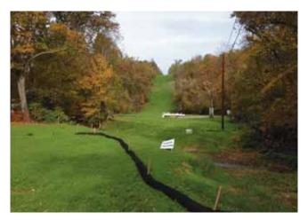
**Figure 4.** EQT pipeline project in Alleghany County, Pennslyvania, on 10/15 after EarthGuard Fiber Matrix was applied.
